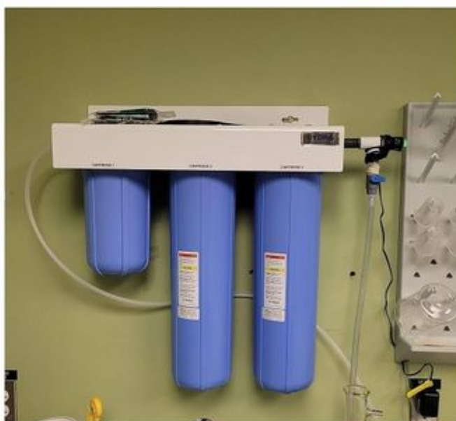
De-ionized water system at PCP WWTP Lab
