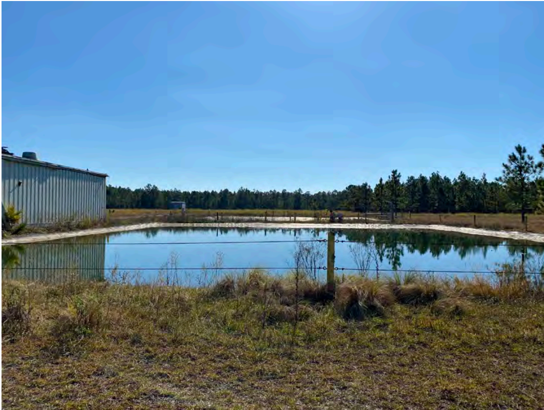
No.3 – WWT1 – Two Lined Wastewater Treatment Ponds - Liners and associated equipment to be removed.
