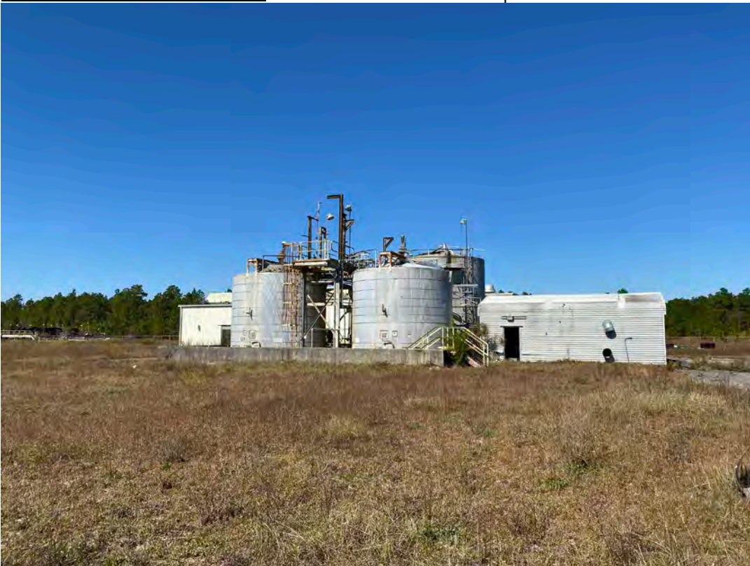
No.12 – Concrete Containment and Tank Farm with Three Steel Insulated Tanks - Entire containment and associated tanks and equipment to be removed.
