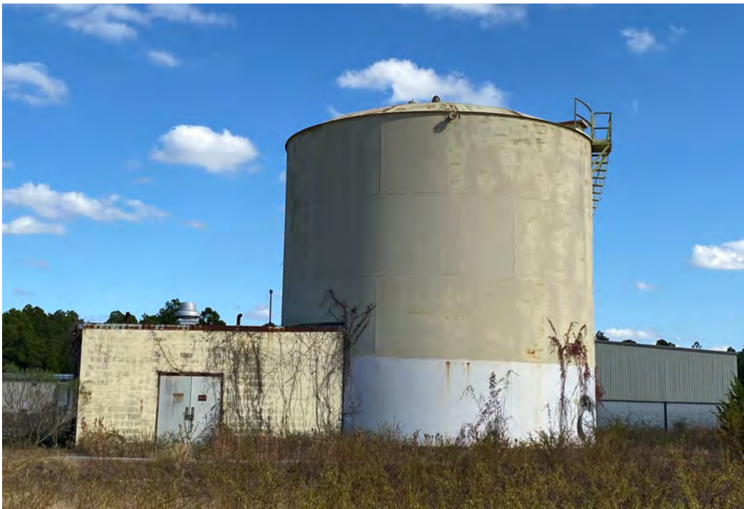
No. 19 - Former Fire Water Tank and Concrete Block Building Entire structure associated equipment, tank and concrete slab to be removed.
