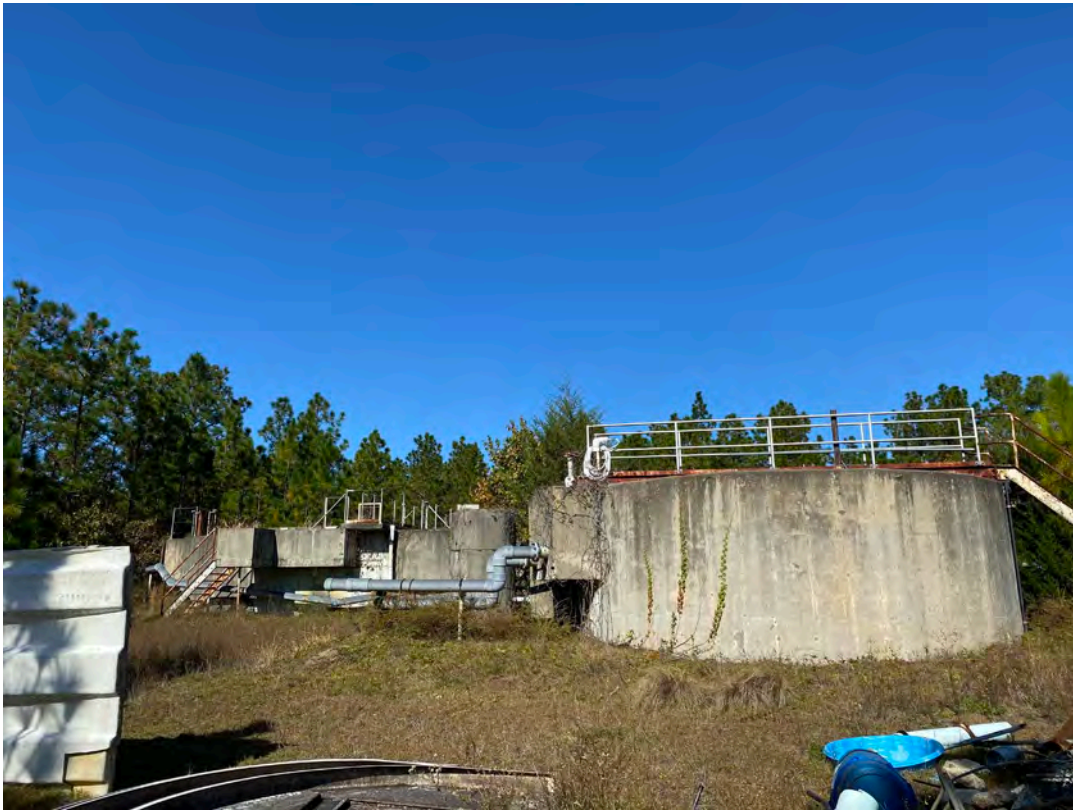
No.5 & 6 WWTI - Rectangular Concrete Oxidation Treatment Tank and Round Concrete Vessel Looking northwest, entire structures and associated equipment to be removed.
