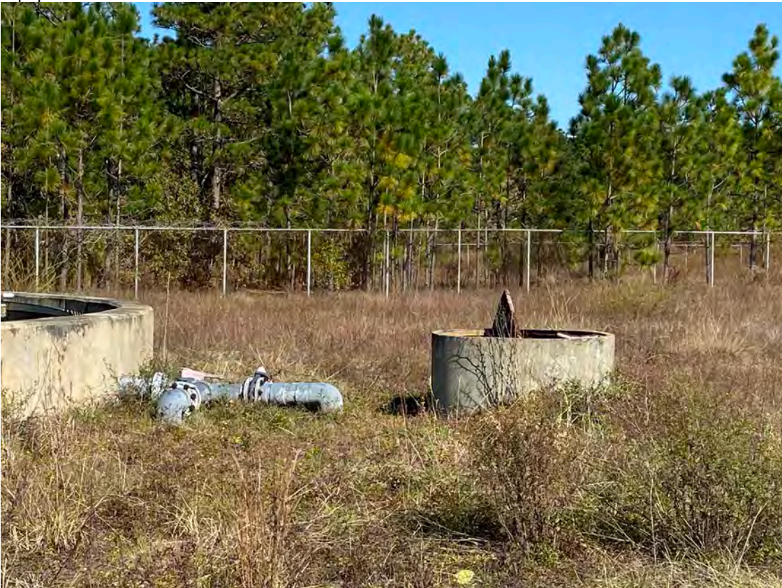
No.2 – WWTI – Approximately 4' Diameter Concrete Sump . Entire structure and associated piping to be removed.
