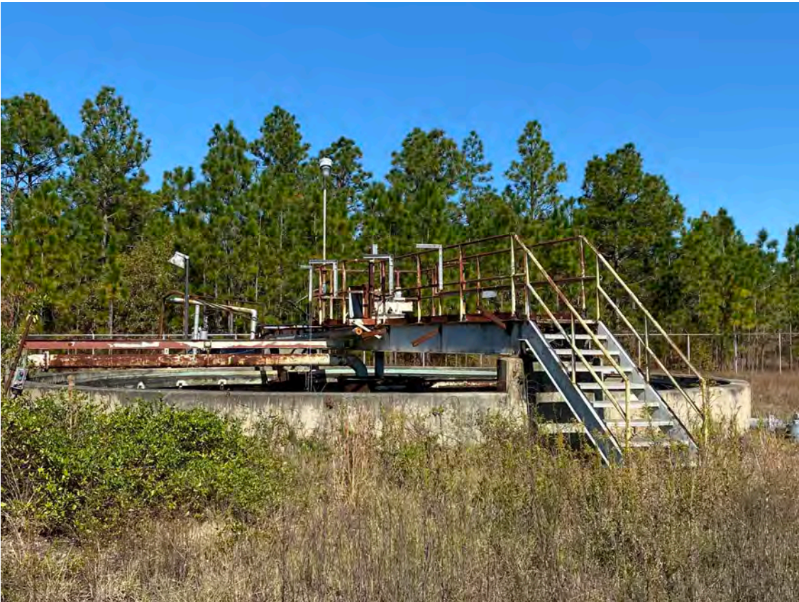
No.1 – WWTI Round Concrete Settling Basin – Entire structure and associated equipment to be removed.
