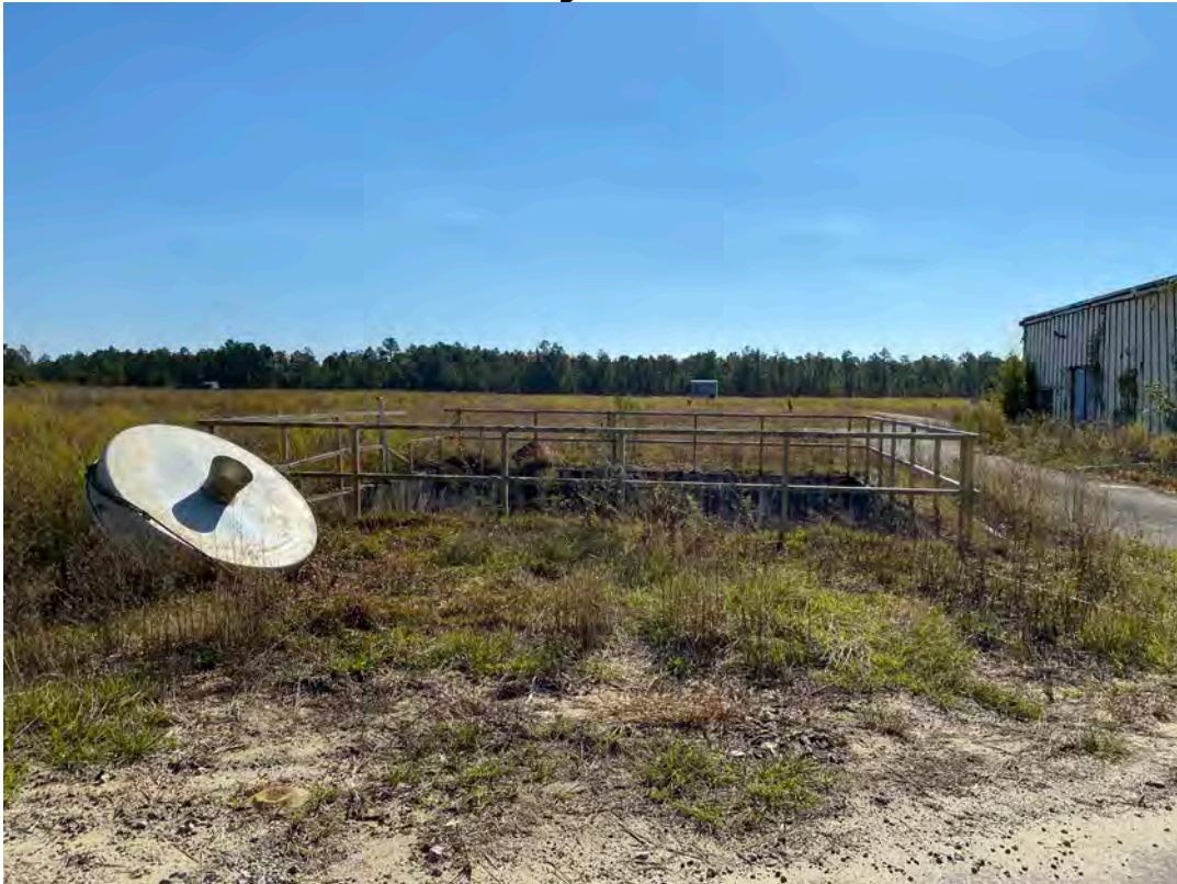
No.8 – Rectangular Concrete Containment with Fiberglass Railing – Entire concrete structure and associated equipment to be removed.
