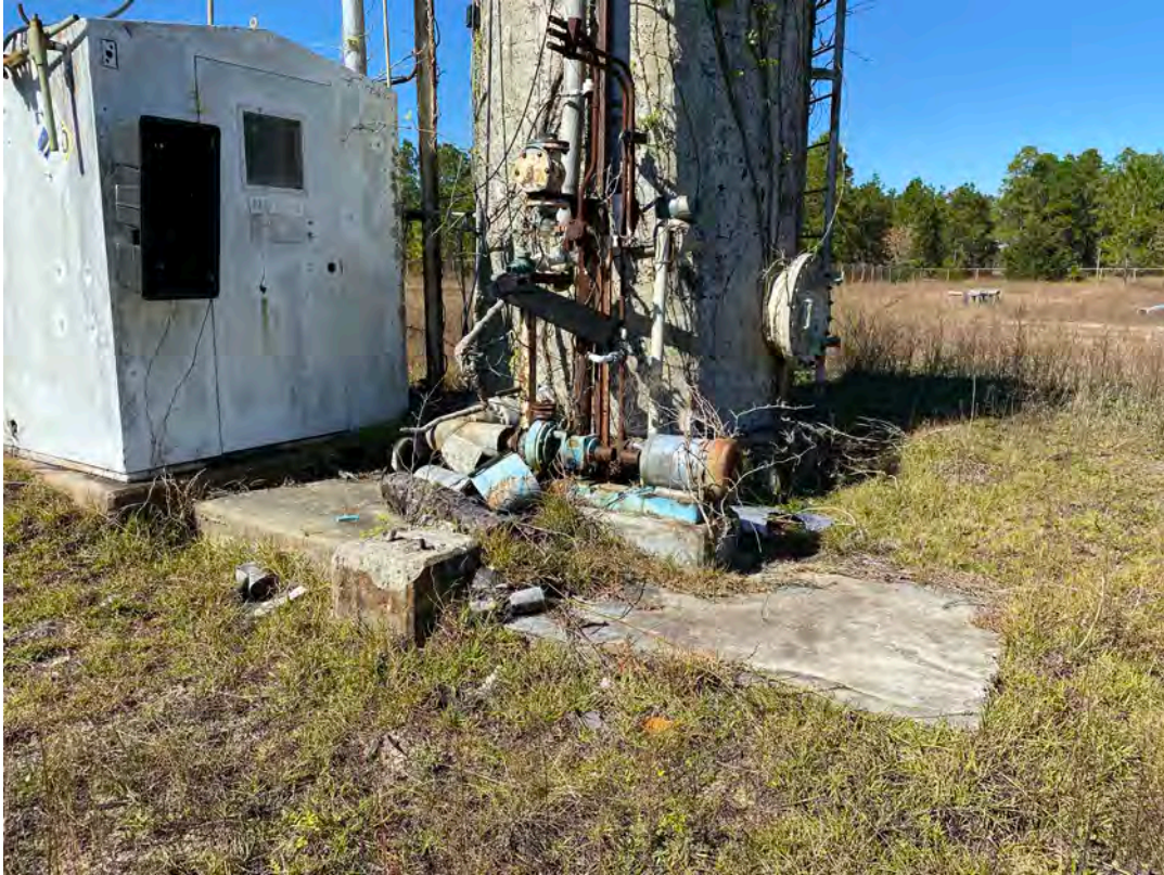
No.15 - Looking Northwest, Sealed Fiberglass Tank and Operators Shed Tank, shed, associated equipment and concrete pad and apron to be removed.
