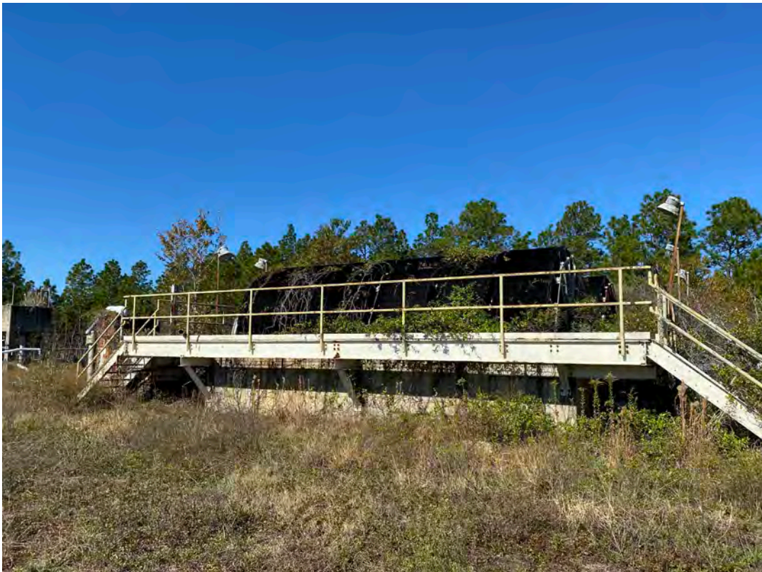
No.4 – WWT1 – Three Rotating Biological Contactors (RBCs) - RBCs entire structure, concrete containment and supporting equipment to be removed.
