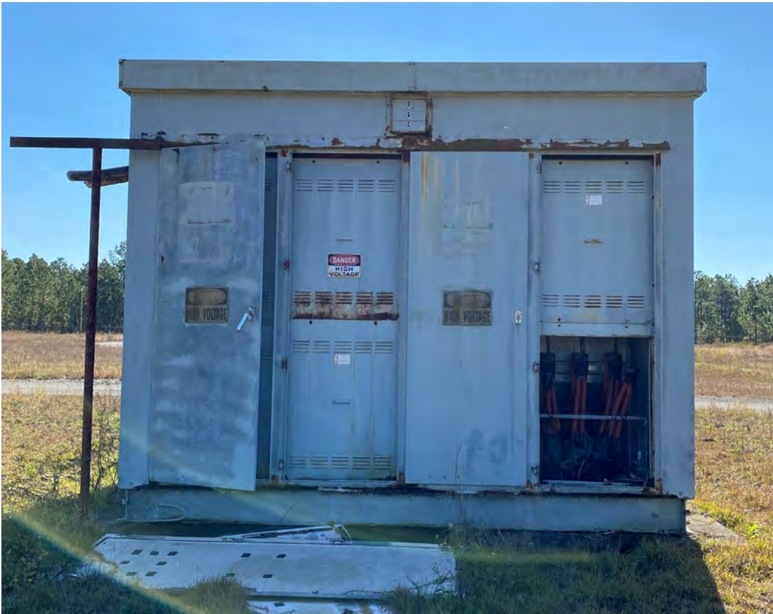
No.11 – Electrical Transformer – Transformer and concrete pad to be removed.
