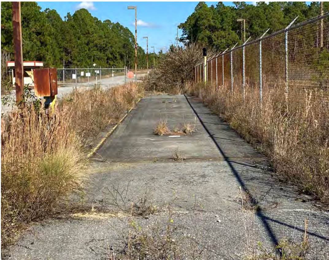
No.24 – Truck Scale – Entire structure and associated components to be removed.
