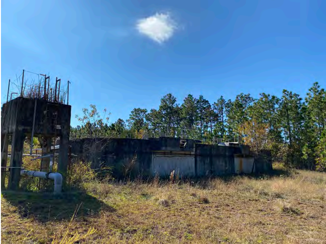
No.5 – WWTI – Rectangular Concrete Oxidation Treatment Tank Looking southwest entire structure, ancillary concrete structure and associated equipment to be removed.
