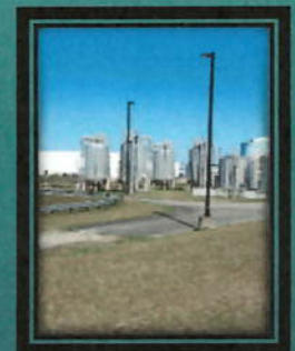
Water Treatment Plant GACs Est. 2012
