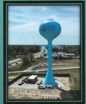
Scotts Hill Elevated Tank Est. 2024
