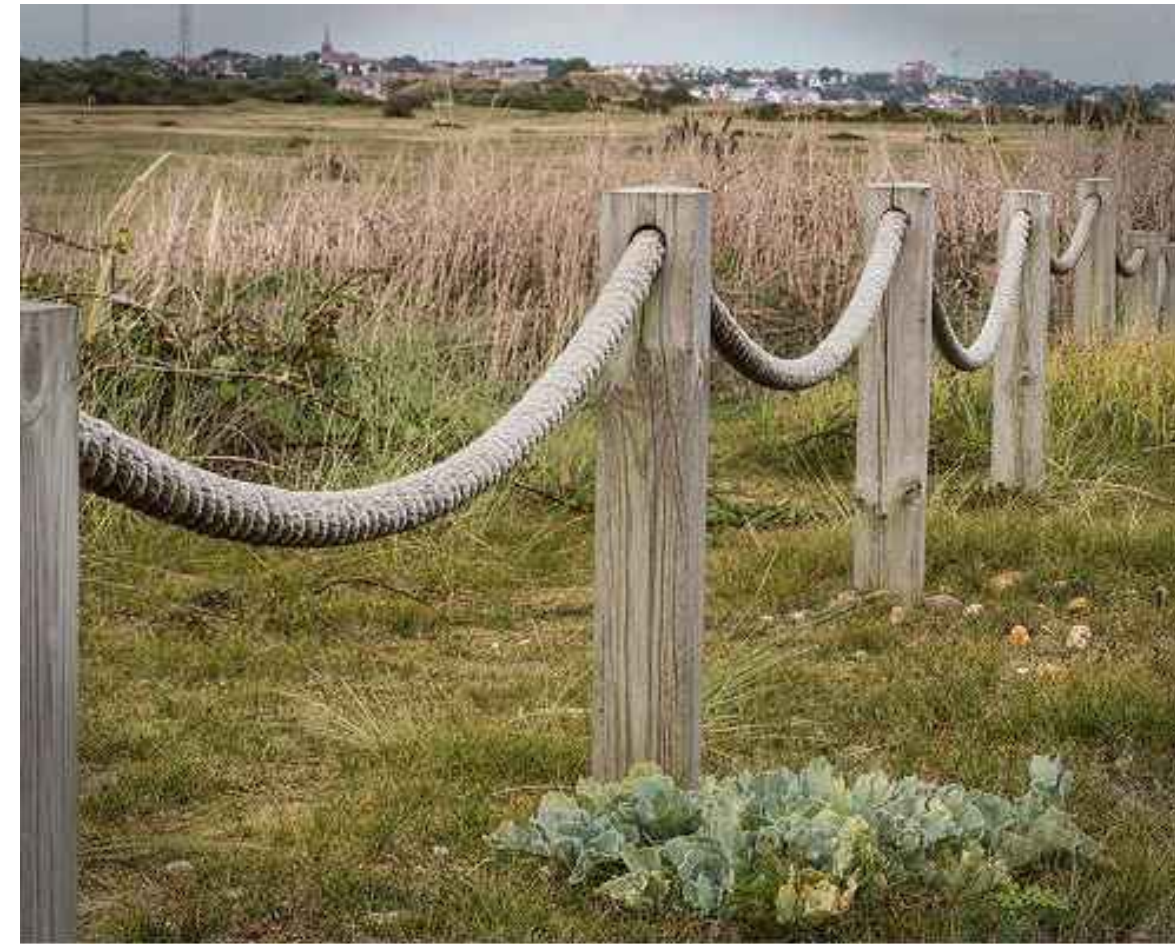
2 WOOD POST AND ROPE BARRIER SCALE: NOT TO SCALE
