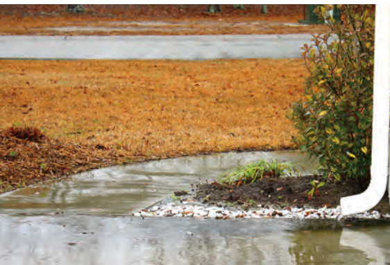
Typical placement of a downspout
